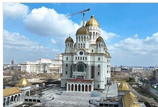
The People's Salvation Cathedral in Bucharest is the tallest and largest Eastern Orthodox church building [b] in the world [269]
